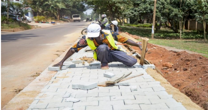
Walkway construction on Ntinda II road
