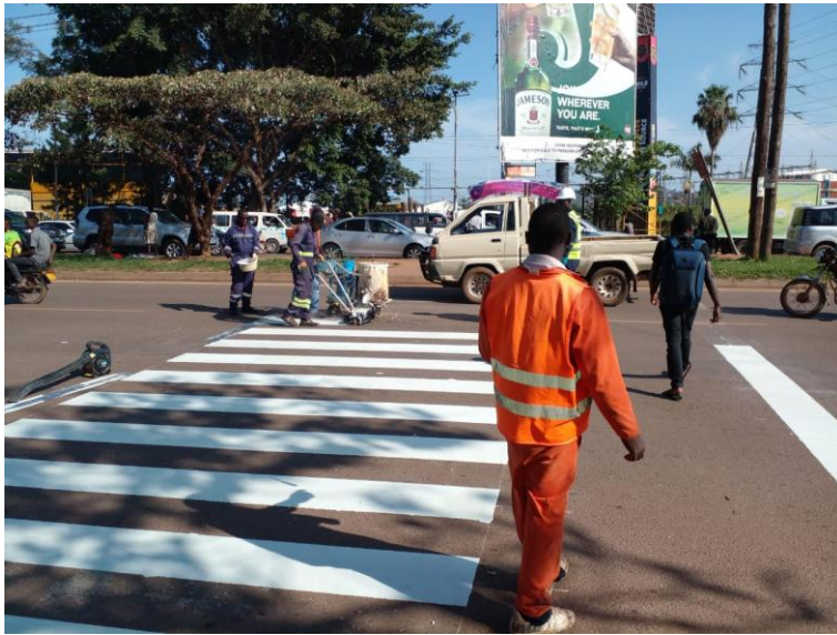
Repainting of faded zebra crossings in the city
